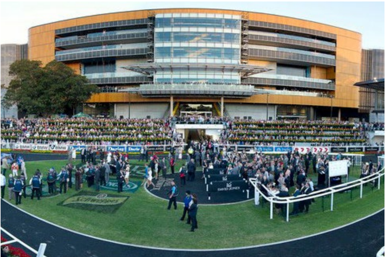
The back of the grandstand at Royal Randwick
